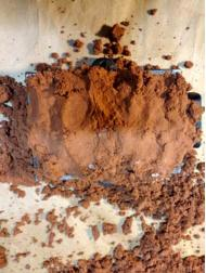
3) Tamp down the sand using a mallet or hammer.
